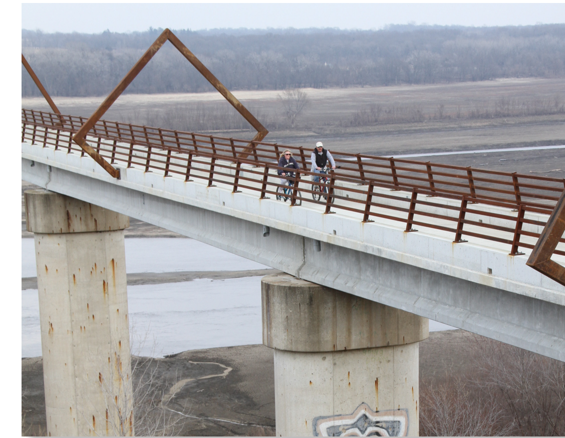
High Trestle Bridge. Source: Mary Swalla Holmes
